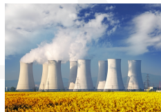
Nuclear Power Generation
