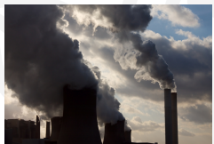
Coal Power Generation
